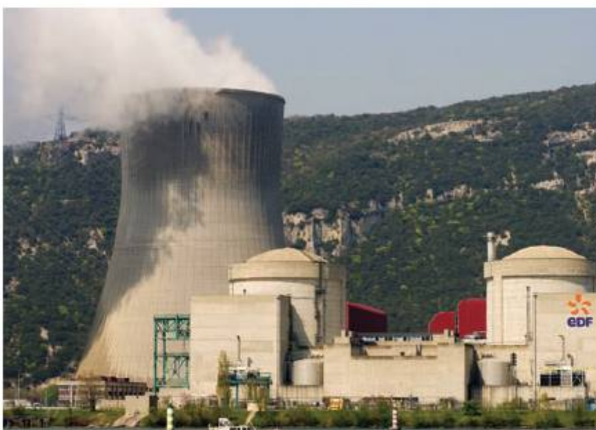
Figure 8.24 The 3.6 GW nuclear power station in Cruas, France, supplies about 5% of the country's electricity needs
