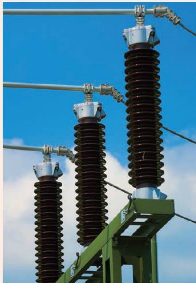
Figure 12.36 Ceramic insulation on a pylon
