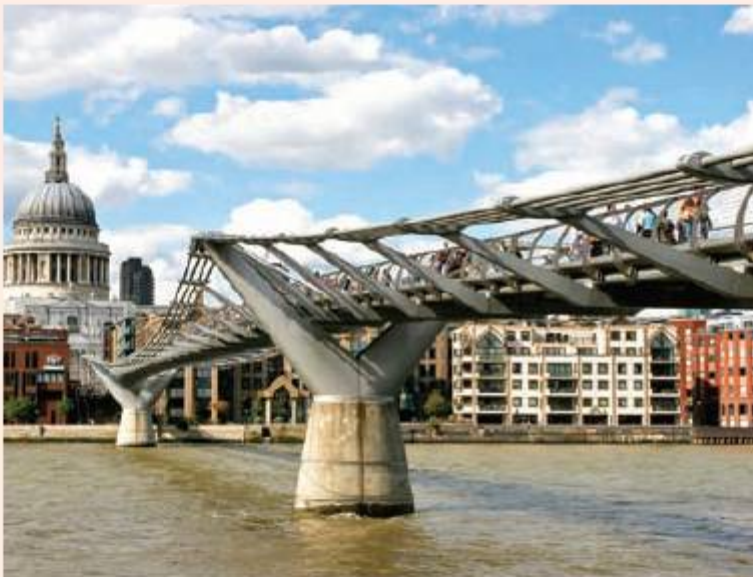
Figure 4.24 The Millennium Bridge in London was affected by resonance
