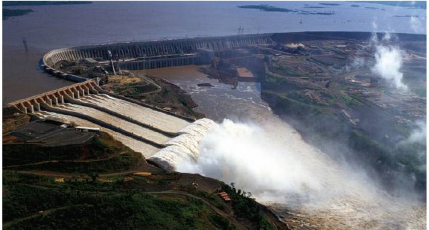
Figure 8.38 The Itaipu hydroelectric power station on the Brazil–Paraguay border
