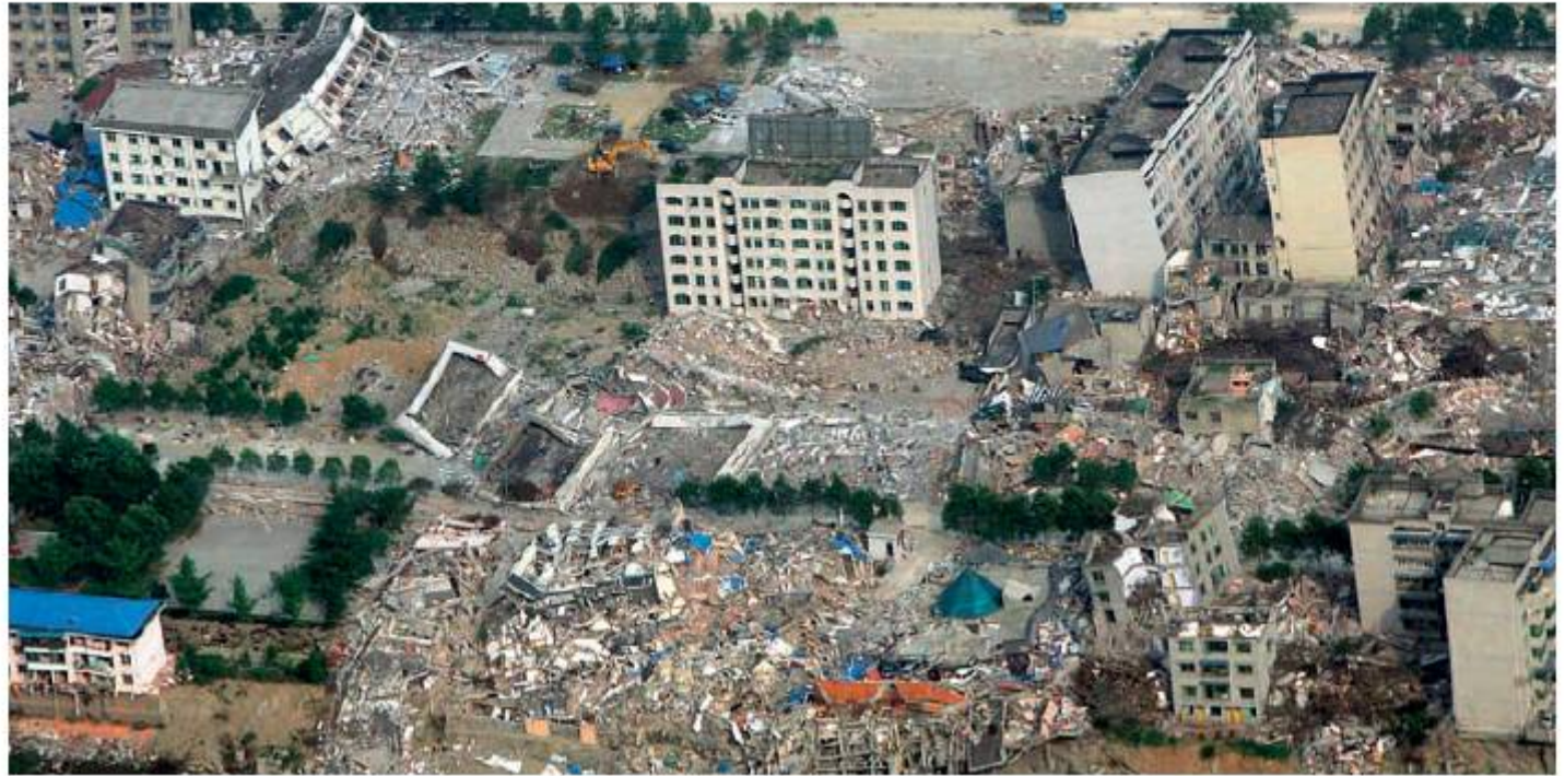
Figure 4.22 Resonance may be one reason why some buildings collapse in an earthquake
