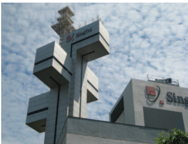
Figure 17.63 SingTel Ayer Rajah Telecommunications Tower, Republic of Singapore
